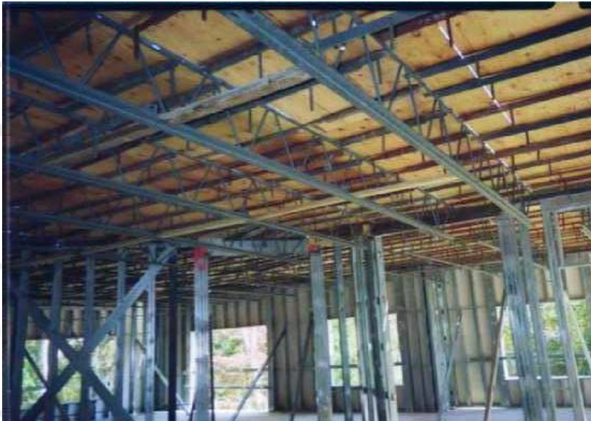
Figure 1: First Floor Hambros Joist Composite Deck System
