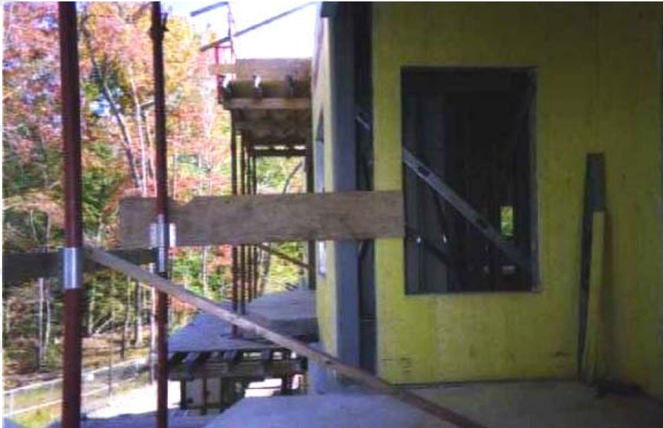
Figure 3: CIP Formwork for Balconies
